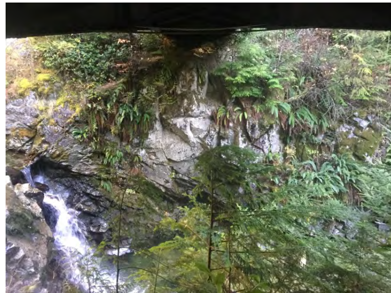
Left Bank Abutment when facing downstream
