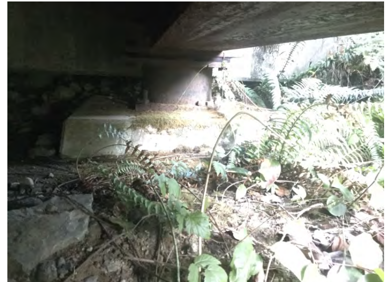
Downstream Left Bank Abutment when facing downstream
