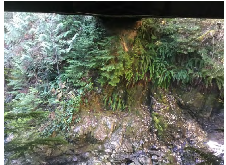
Right Bank Abutment when facing downstream
